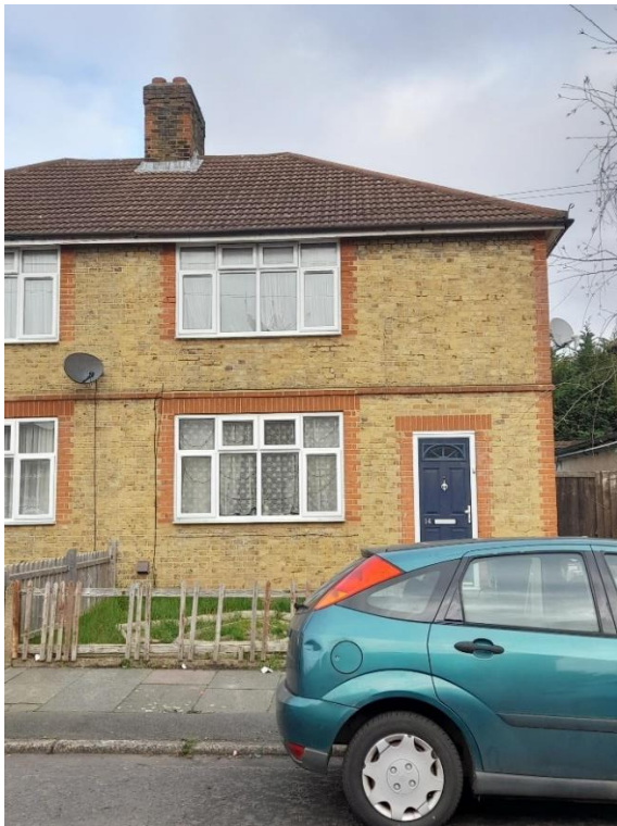
- Home before works began
