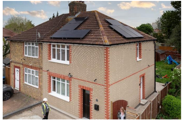
- Completed retrofitted home including solar
